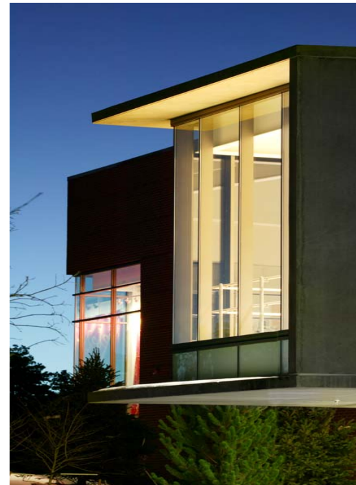
Kent Denver Center for the Arts Englewood, Colorado Architect: Semple Brown Design
